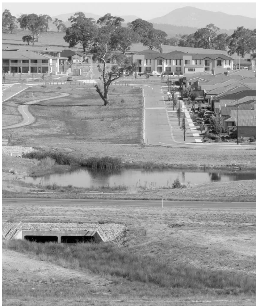
Fig. 6. Example of a typical under-road box culvert along a natural drainage line in the Gungahlin suburbs.
